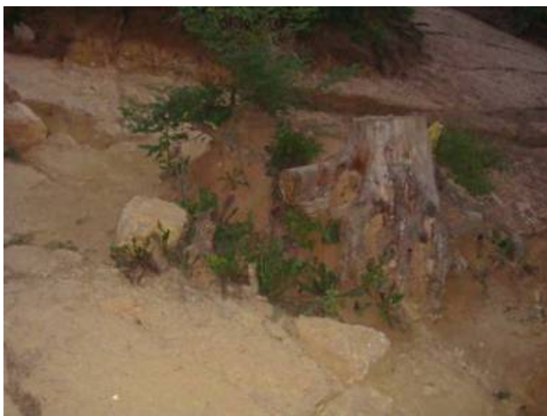
Photo 36: Tree roots can not permeate the cement surface of the Pyramid. According to the biologist professor Sulejman Redzic of Univesity of Sarajevo, same roots break through natural conglomerate material for 20-25 meters (Neretva river valley, 120 km south of Visoko)
