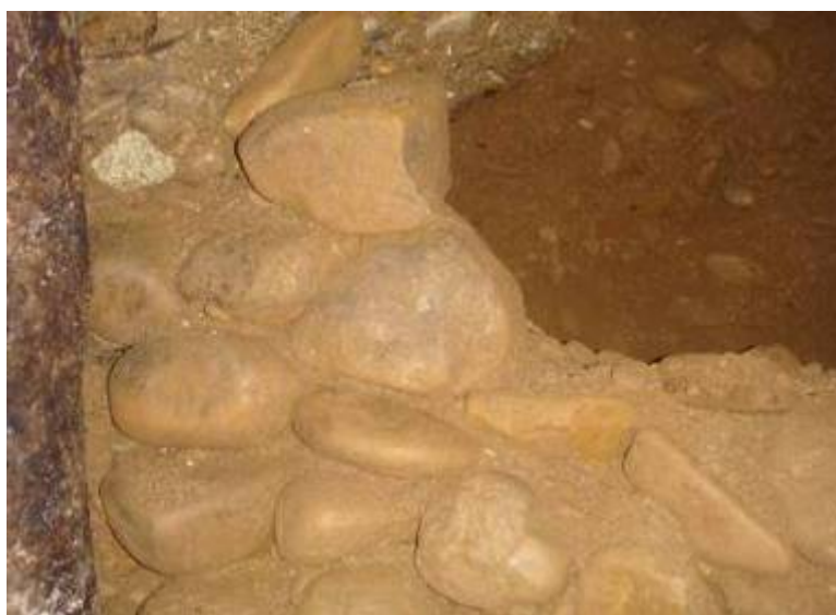
Photo 61: Drywall detail in underground tunnel complex “Ravne” (70 meters from the entrance).
