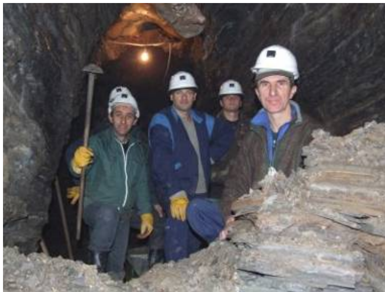
Photo 70: Discovery and cleaning of the debris in the underground tunnel “KTK”; October 2007 – February 2008. Tunnel was 3 meters high and 2.5 meters wide.
