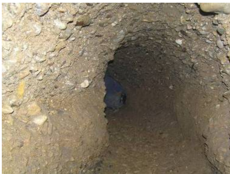
Photo 58: Size of underground tunnel “Ravne” at the time of discovery in 2006. Tunnels are built in conglomerate material. Approx. 50 cm of conglomerate layers are above the marl material (water-tight). Tunnel complex was flooded in distant past and lot of debris remained.
